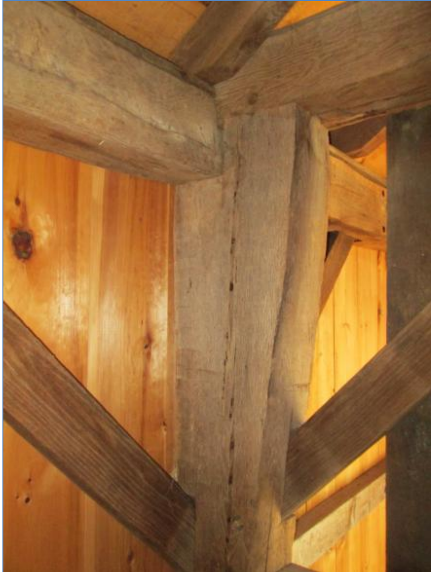
Gunstock post/joinery in the Brunn Barn
