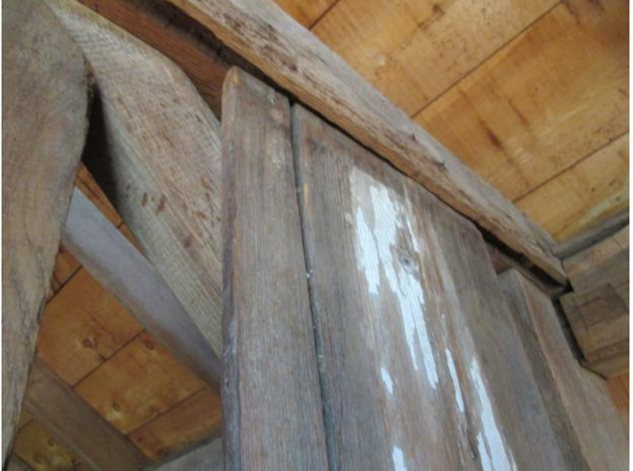
Beam is grooved to accept tops of sidewall boards
